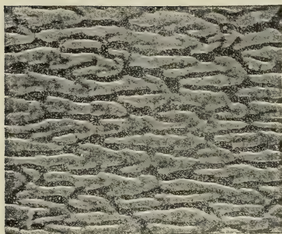
FIG. 122.—Prepared Roofing Finished in a Veined Surface.
